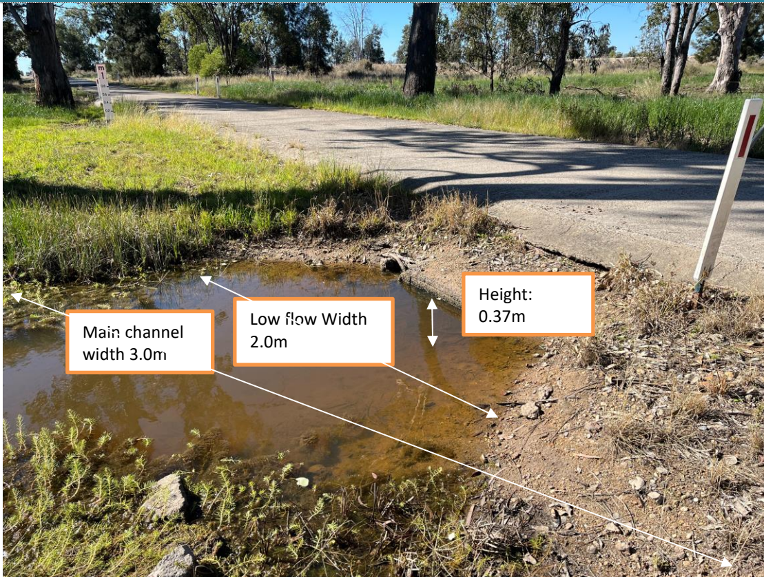
Smaller culvert on upstream (western) side of bridge
