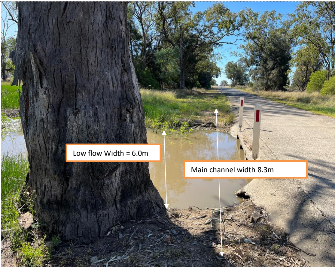
Larger culvert on upstream (western) side of bridge
