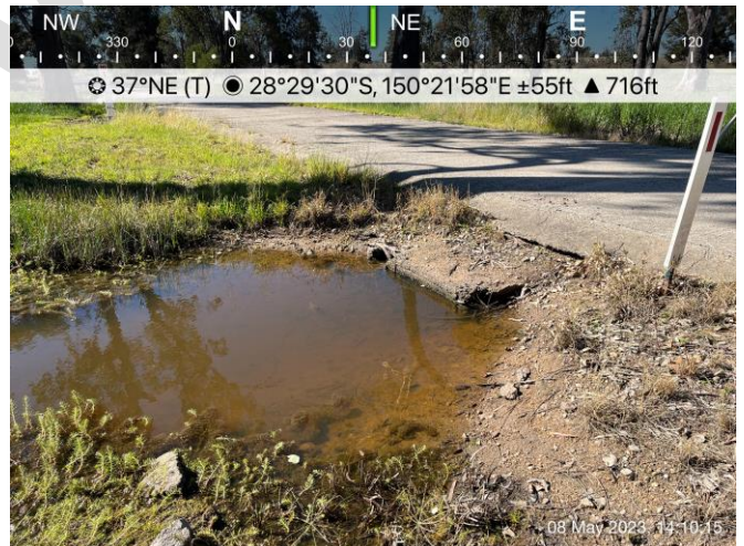
Small pipe just south of the culvert on the floodway
