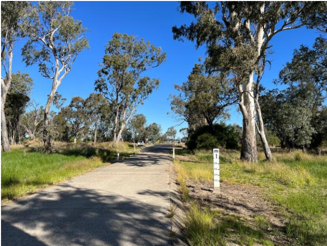
Culvert crossing looking south toward Cunningham Highway
