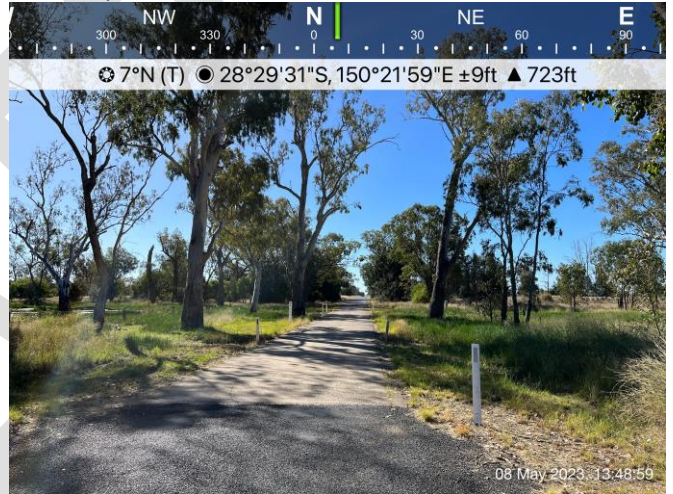
Culvert crossing looking north
