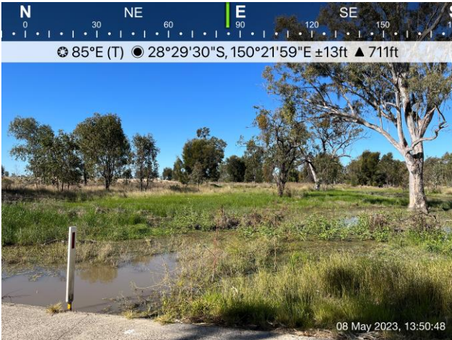
Landscape in eastern direction from culvert
