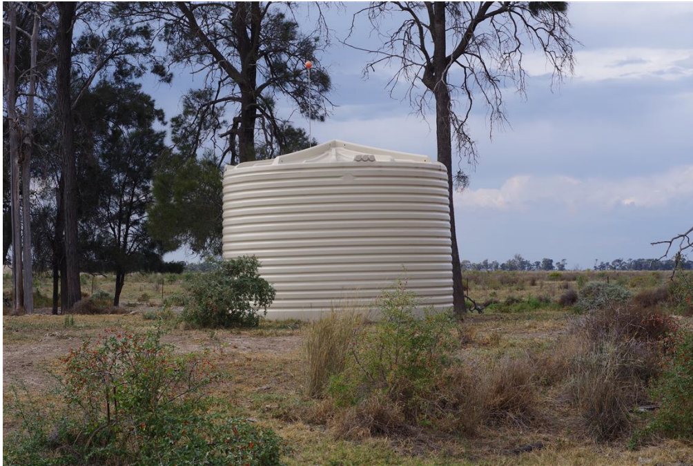
Figure 6.3 Existing water tank on Gunsynd SF.
